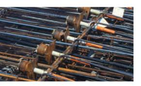
Prestressing by post-tensioning, as opposed to bonded wires tensioned before the concrete is poured, comes in two types:
