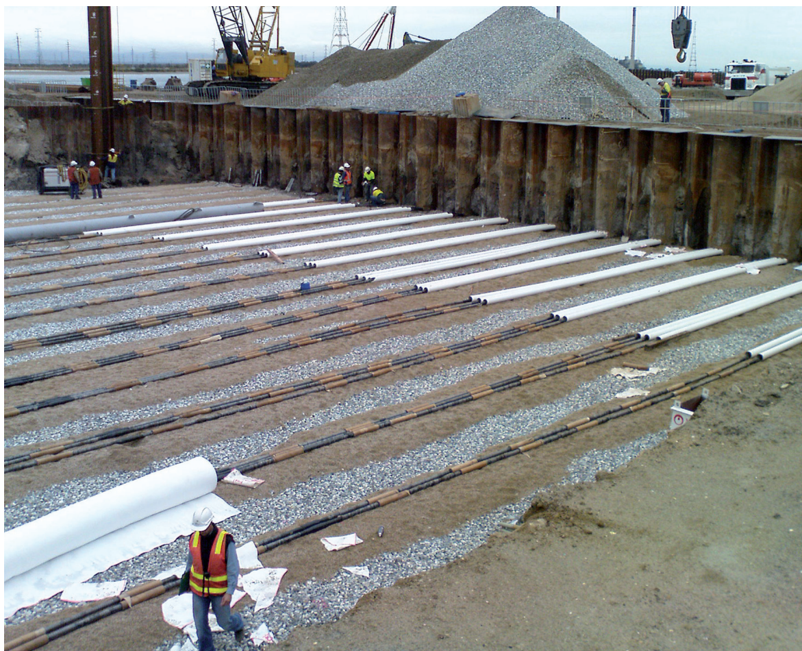
Permanent ties for quay walls
