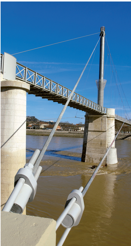
Anchorage of steel ropes
