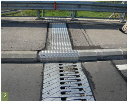
1. Installation of an NFT joint 2. NFT joint seam and footpath adaptation
