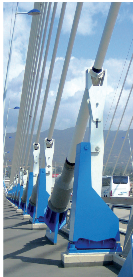
PED damper Charilaos Trikoupis bridge / Greece
