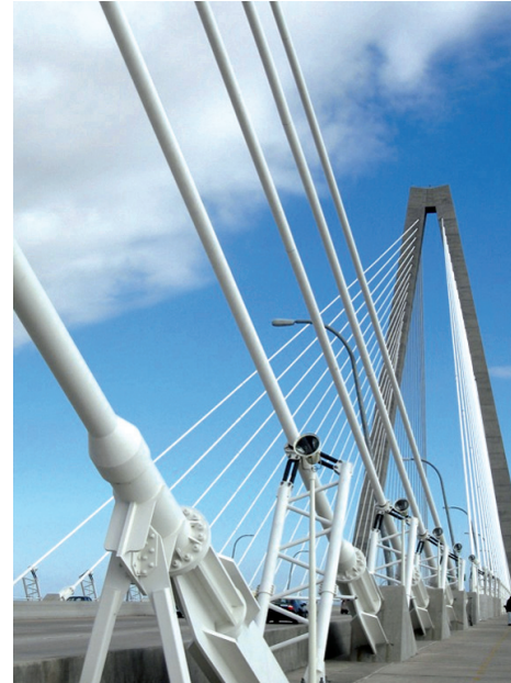
FED damper Cooper bridge / USA
