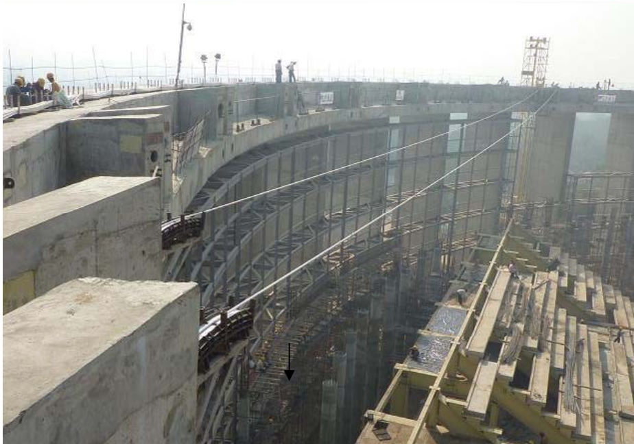
Initial ref. strand launching and adjustment (sag)
