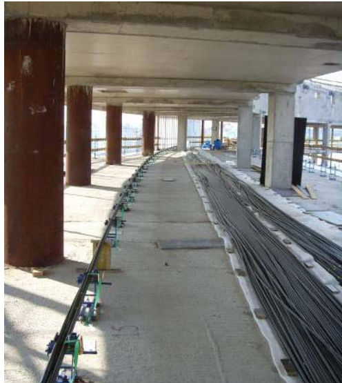
Prefabrication bench
