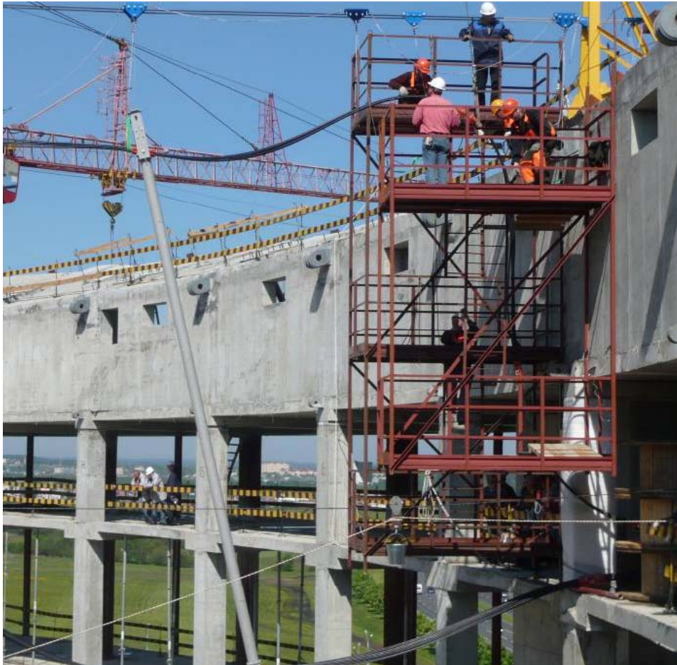
Cable launchin with mast installation
